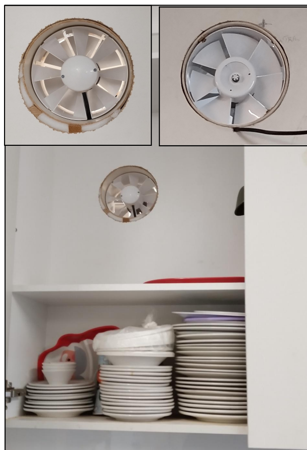
The Pressurising Fan in the Kitchen Crockery Cupboard.
